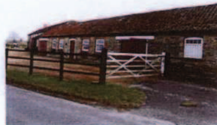
Single storey Farm Buildings
