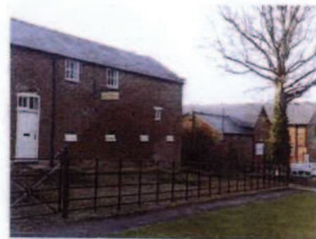
Buildings further along Langton Road
