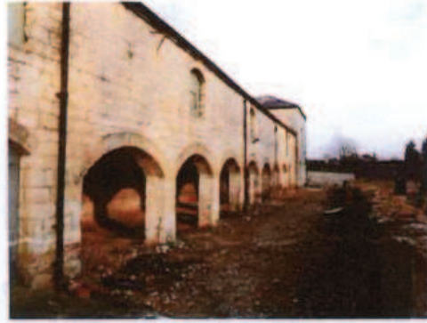
The Listed Barn next to the site
