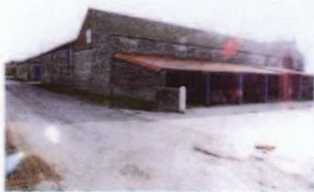
Barns with lean-to sheds
