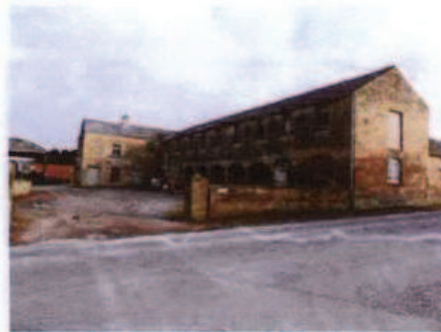
Estate Buildings at Birdsall
